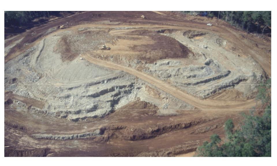
Mine Operations; Annual Ore Production Target 750,000 Wet Metric Tons Ore. 35 ton excavators, D8 Dozers, 40t 6x6 Articulated Trucks, 6x8 Trucks. 14H Grader. Free Dig Operation.
